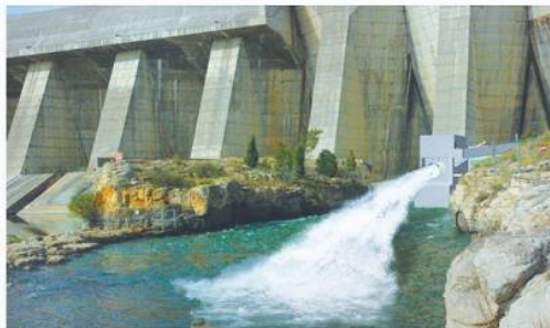
The Southern Delivery System will collect raw water from the reservoir impounded by Pueblo Dam, on the Arkansas River, and deliver it to Colorado Springs, Colorado. A new connection to the existing river outlet works will divert a portion of the flow to the pipeline via a valve structure on a platform to be erected in the river. The remainder of the water will discharge to the river.
