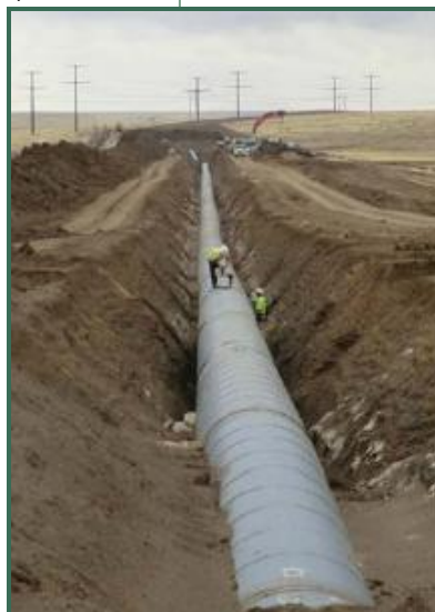
Work continues at North Pipeline 1A
