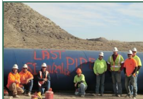
Last pipe installed at South Pipeline 1
