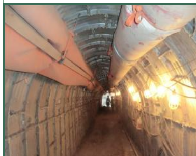
Tunneling under the Union Pacific Railroad on South Pipeline 1
