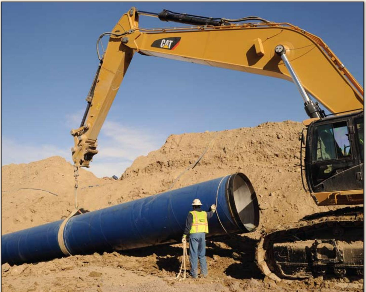
**66" diameter polyurethane coated and cement-mortar-lined steel water pipe produced to AWWA standards from American steel by the Northwest Pipe Company for the SDS project.**
