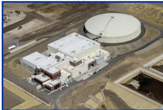
Edward W. Bailey Water Treatment Plant
