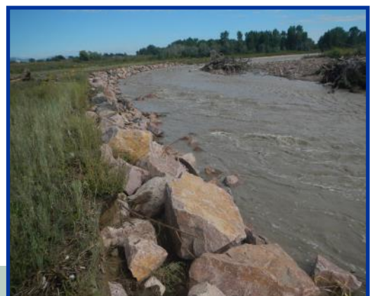
Improved grade control work along Fountain Creek
