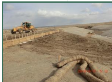
Revegetation on South Pipeline 3
