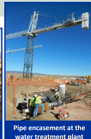
Installation of rebar at the water treatment plant
