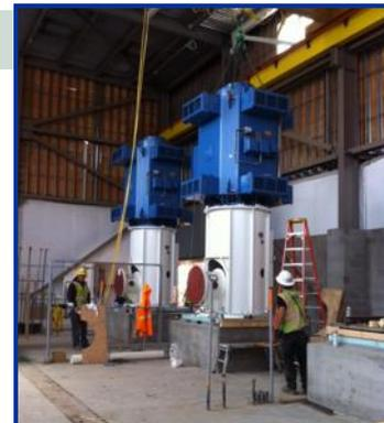
Installation of pumps and motors at Juniper Pump Station
