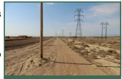
Trail improvements at South Pipeline 2
