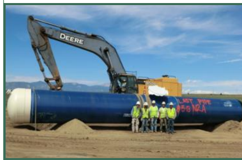
Last pipe for installation on North Pipeline 2A
