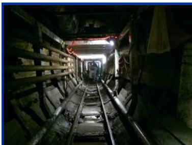
Progression of tunnel excavation for South Pipeline 4A Central
