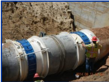
Installation of 60-inch diameter filter effluent pipe
