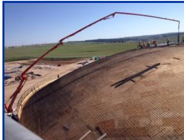
First dome concrete pour for the raw water storage tank
