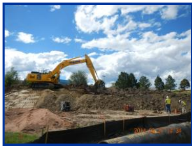
Restoring berm on west side of Powers Blvd. for Finished Water 3
