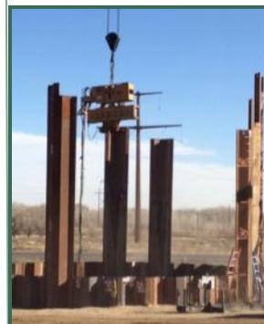
Driving sheet piles at South Pipeline 4A Central
