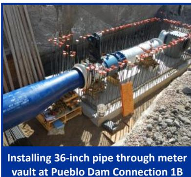
Installing 36-inch pipe through meter vault at Pueblo Dam Connection 1B
