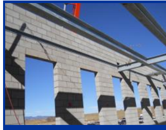
Installation of structural steel
