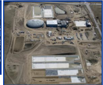
Aerial of the water treatment plant
