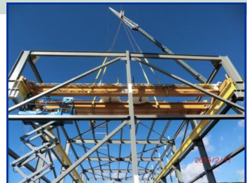
Setting bridge crane at Bradley Pump Station
