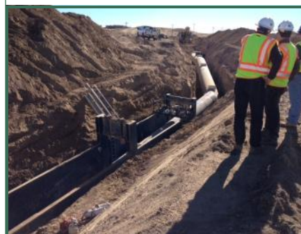
Pipe installation at South Pipeline 4A West
