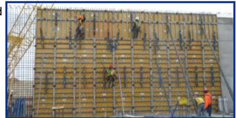
Wall form installation for a structure at the water treatment plant
