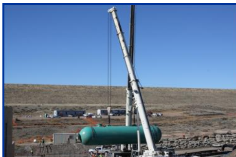
Setting surge tank at Juniper Pump Station
