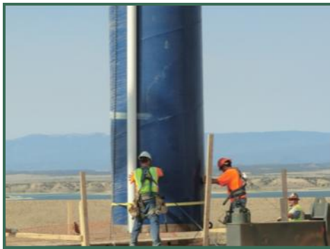
Installing shaft riser pipe at South Pipeline 1
