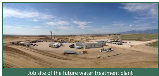
Job site of the future water treatment plant
