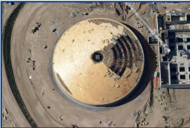
Construction of the raw water storage tank dome
