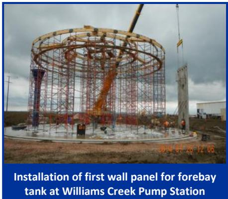
Installation of first wall panel for forebay tank at Williams Creek Pump Station
