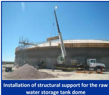
Installation of structural support for the raw water storage tank dome
