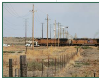
Overhead wire crossing at Williams Creek Pump Station power supply
