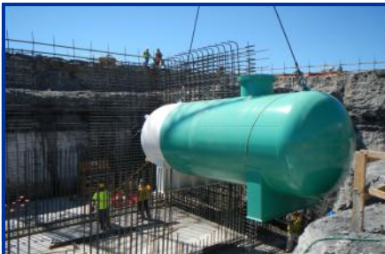
Installation of the surge tank strainer vault at Juniper Pump Station
