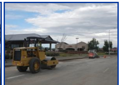
Paving operations at Powers Blvd. and New Center Pt.
