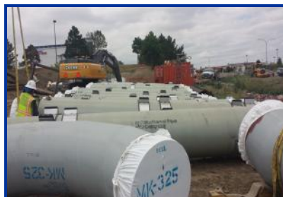
Pipe for Powers Blvd. tunnel
