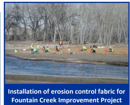
Installation of erosion control fabric for Fountain Creek Improvement Project
