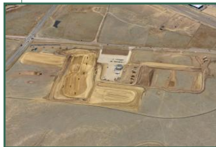
Aerial view of the water treatment plant
