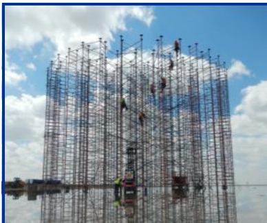
Crews building temporary support for the raw water tank concrete dome
