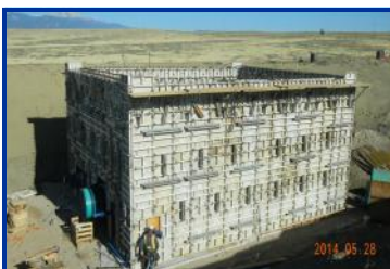
Forming walls for discharge valve vault at Bradley Pump Station
