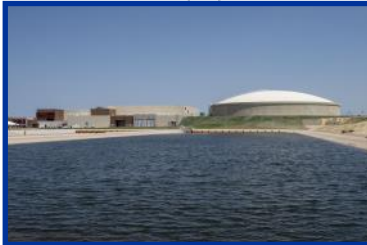
Edward W. Bailey Water Treatment Plant
