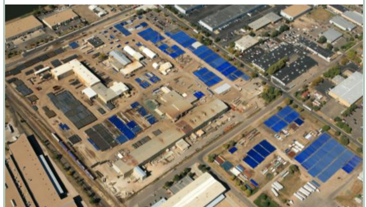
Aerial view of pipe fabricated for SDS by Northwest Pipe in Denver (blue-coated and uncoated pipe is all for SDS), October 2011
