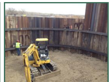
Inside the launch shaft at South Pipeline 4A Central
