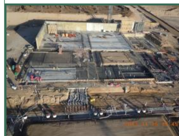
Aerial view of construction at the water treatment plant
