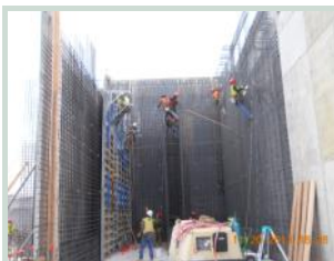
Installation of rebar at the finished water pump station
