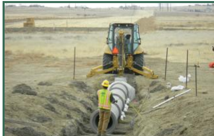
Drainage pond outlet pipe at Bradley Pump Station
