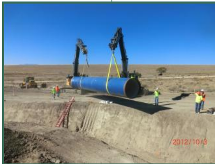
Installing pipe in trench at South Pipeline 1
