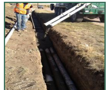
Placement of electrical ductbank for Bradley Pump Station Power Supply
