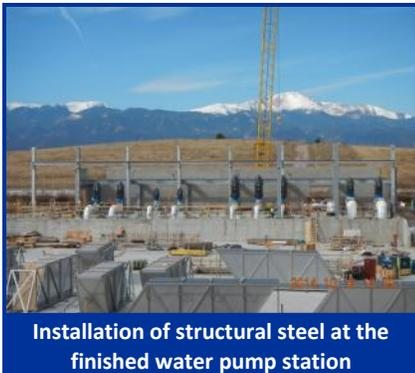
Installation of structural steel at the finished water pump station
