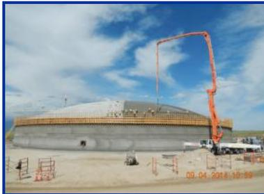
Placement of concrete at the raw water storage tank
