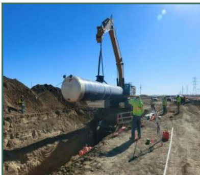
Delivering and laying pipe for South Pipeline 2
