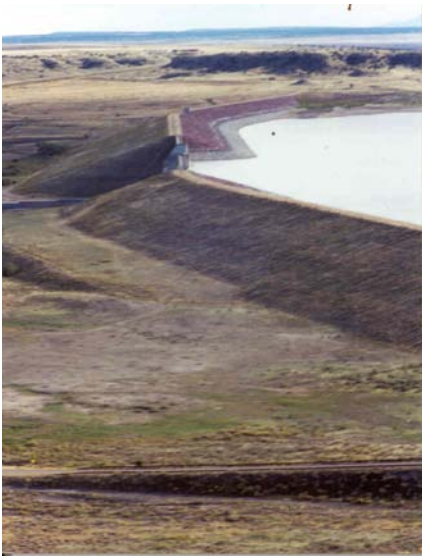
The long earthen embankment at Pueblo Dam
