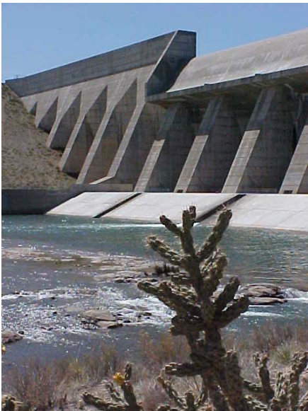
The concrete spillway at Pueblo Dam
